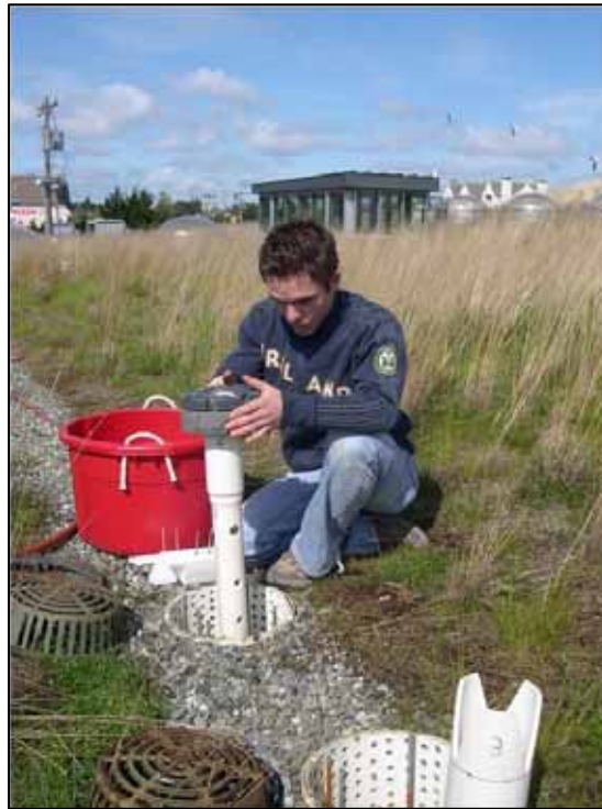
Figure 2-8 Installation of the V-notch Weirs for Monitoring Bypass Flows in the Roof Drain
