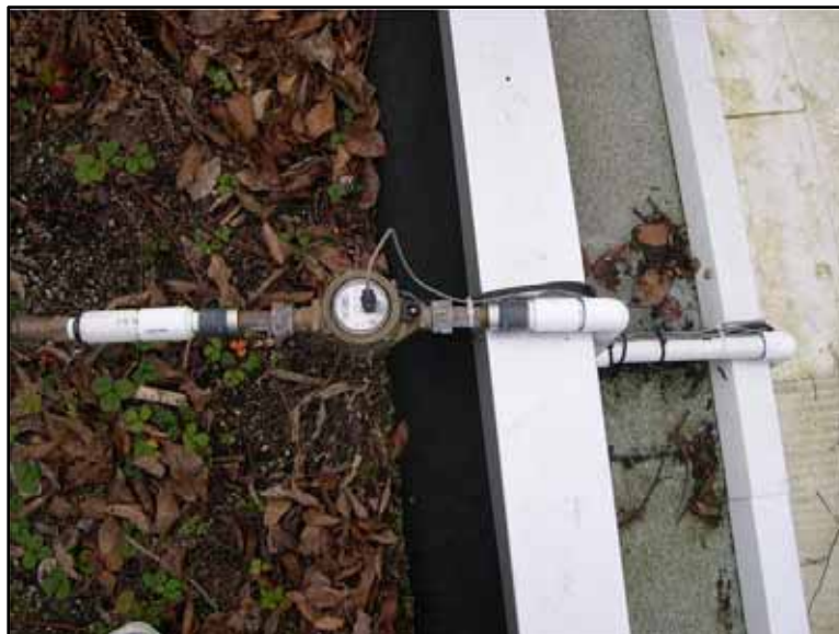
Figure 2-15 Multijet Meter Installed for Measurement of Irrigation Water Delivered to the Ross Park Shelterhouse green roof
