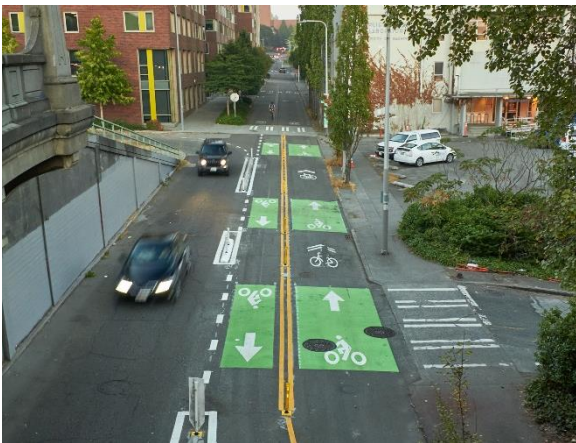
New protected bicycle lane buffer on NE 40th St.
