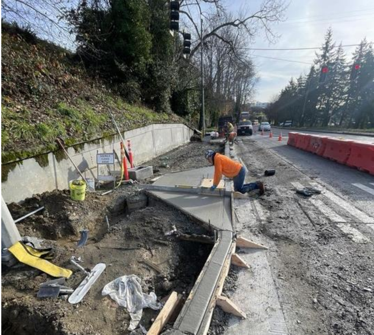
Crews installing curbs and curb ramps on the east side of MLK Jr Way S and S Bayview St as part of the MLK Jr Way Safety Project.
