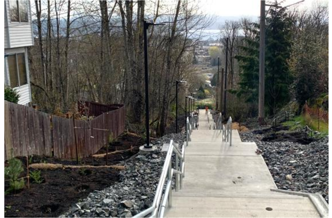
New stairway at S Henderson St.
