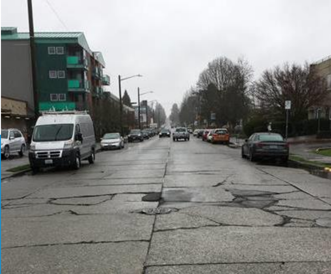
44 th Ave SW - Before
