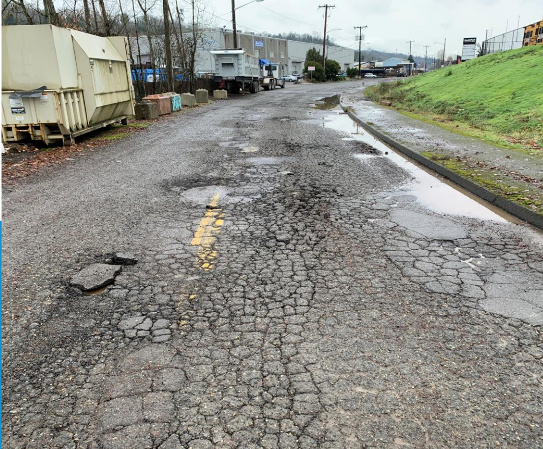
Occidental Ave S - Before
